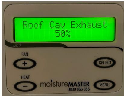
In the **50%** position the Roof Cavity Exhaust damper is only closed half way and therefore approximately 50% of the exhaust air will come from the roof cavity with the remaining 50% being exhausted from within the home.
