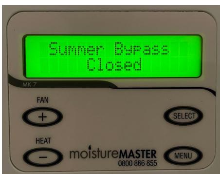
When the **Bypass is Closed** all the fresh air from outside passes through the heat exchange system.
