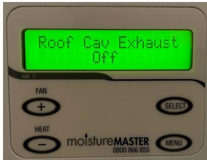
In the **Off** position the Roof Cavity Exhaust damper is fully closed and all of the exhaust air is sourced from inside the home.
