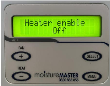
If the Heater enable is off the heater will not operate and the temperature of the source air will only reflect the air temperature that the exchange plate is capable of delivering to the supply side of the system to the house.
