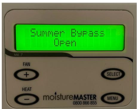
When the Bypass is Open all the fresh air from outside bypasses the heat exchange system and travels directly to the inside.
