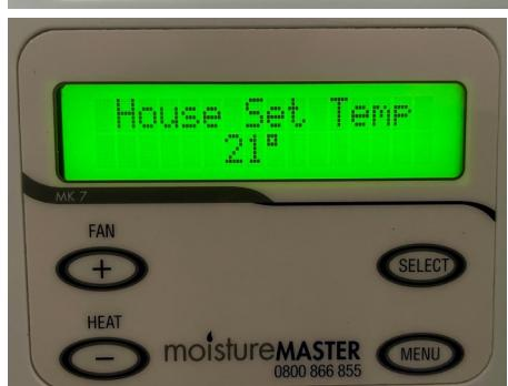
When there is not enough heat within the home to deliver the Set House Temperature from the HX unit the booster heater will deliver this temperature if the Heater is "enable".
