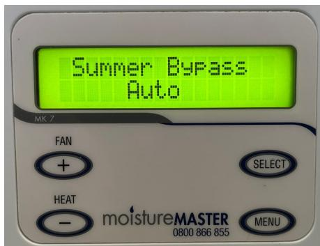
In the **Summer Bypass Auto mode** the system switches from closed to open at selected temperatures in the installer set-up. These temperatures can only be changed in the "Installer Set – Up",
