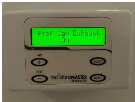
In the **On** position the Roof Cavity Exhaust damper is fully open and sources all of the exhaust air from the roof cavity.
